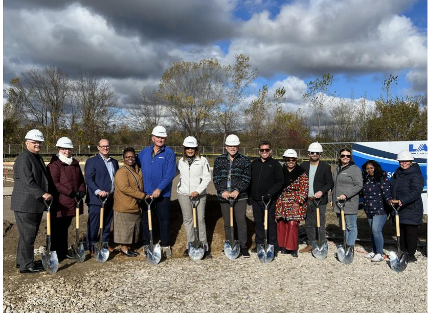
The LAFCU team celebrates the start of construction on the Perry ITM/ATM site, part of the credit union's continued commitment to serving members where they live and work.
